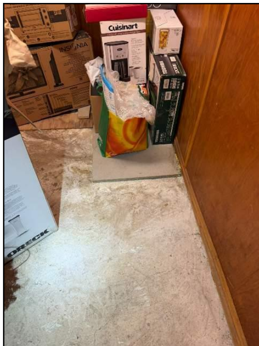
77. Efflorescence
