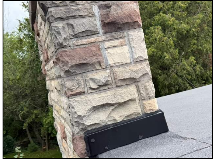
9. Not let into mortar joints
