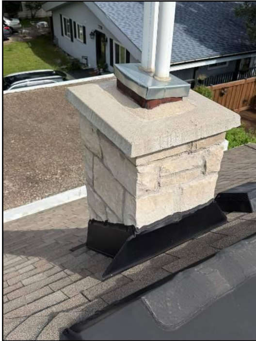
8. Not let into mortar joints
