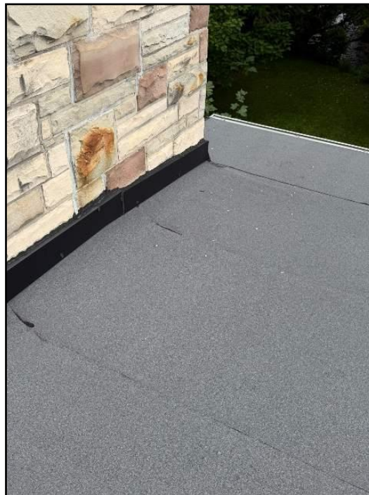
4. Modified bitumen membrane
