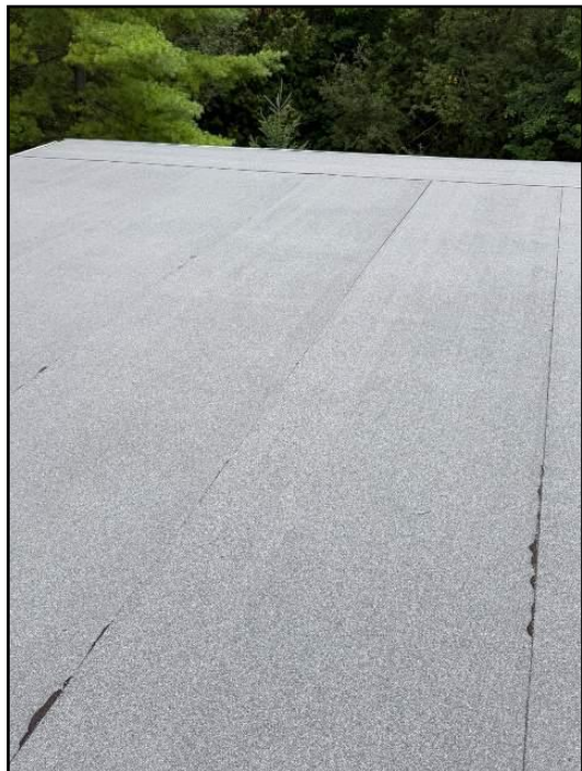
3. Modified bitumen membrane
